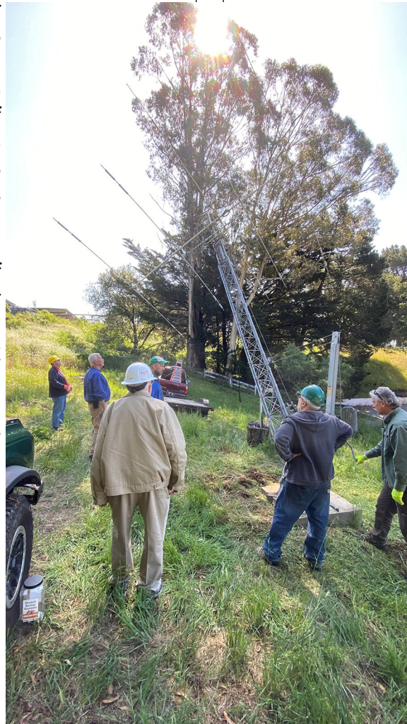
Fig. 1 — Lowering the Tower
