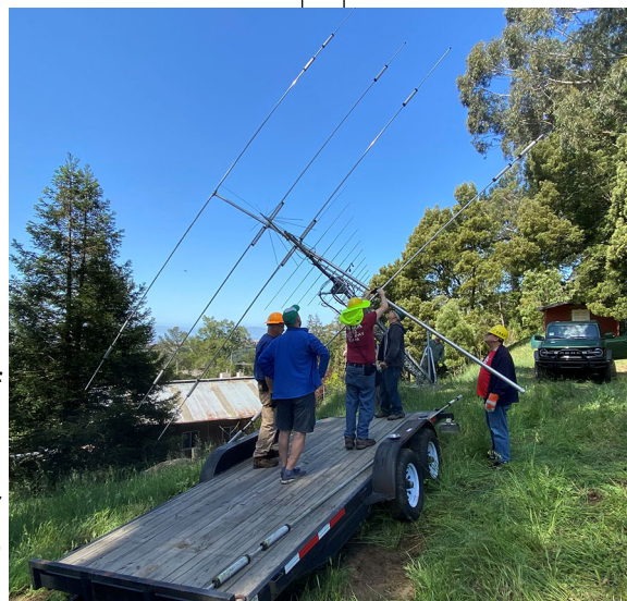
Fig. 2 — Removing the Antennas
