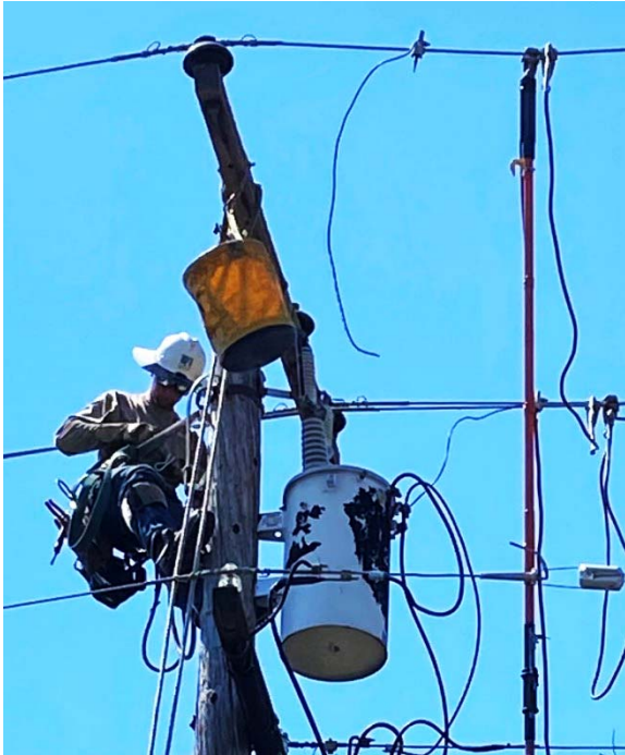
Fig. 5 PG&E Lineman working on insulator replacement – permission from PG&E workman
