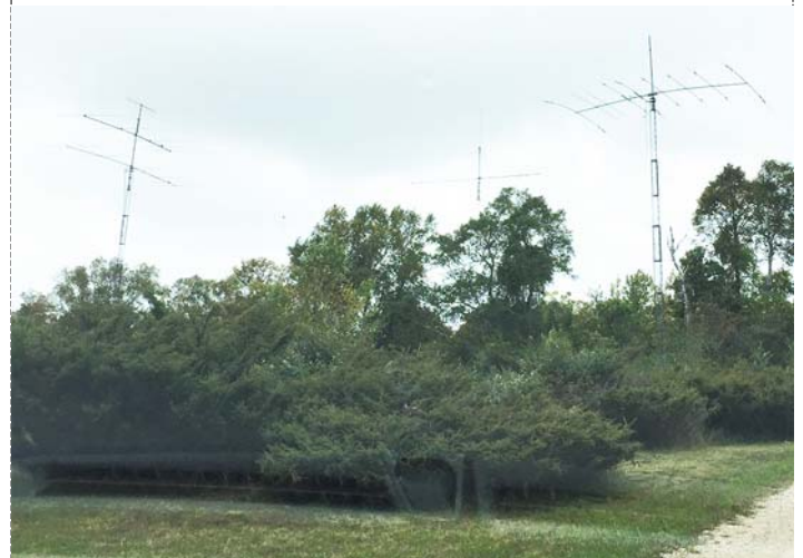
Fig. 5 - Antenna Farm Replacing Orchard
