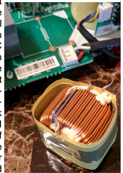
Coil next to power supply board before repair
