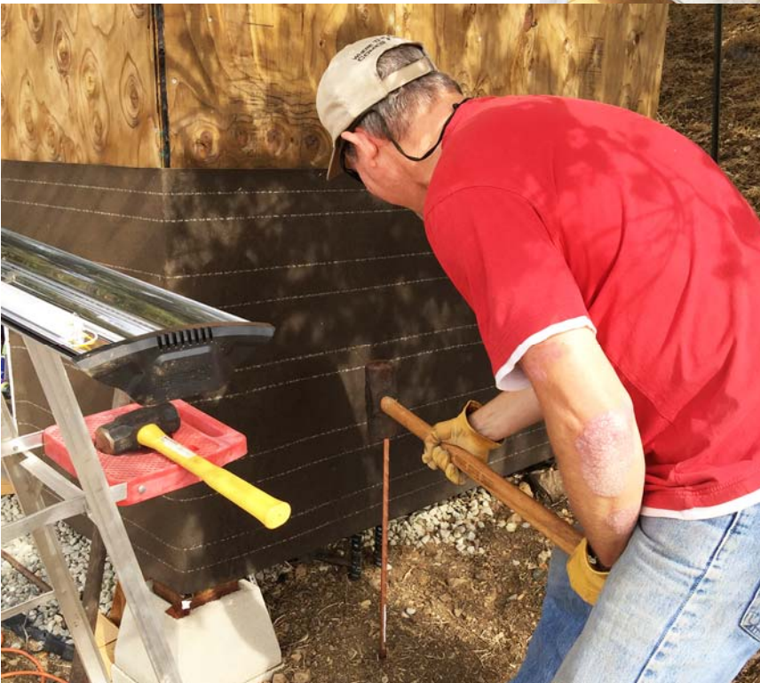
Joel KD6W driving a ground rod
