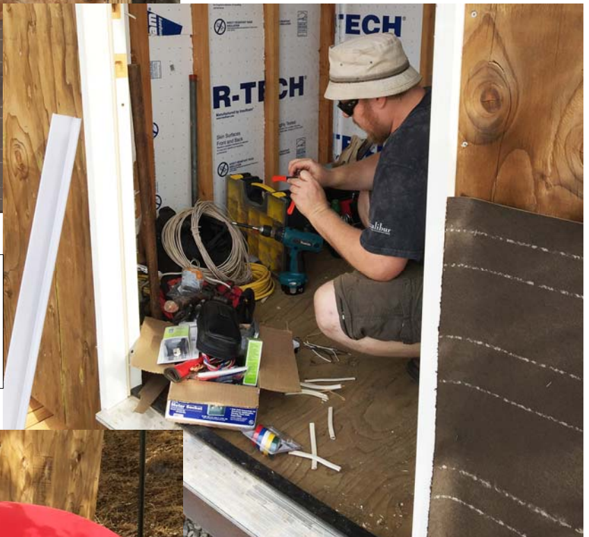
Eric KI6LAY installing an outlet
