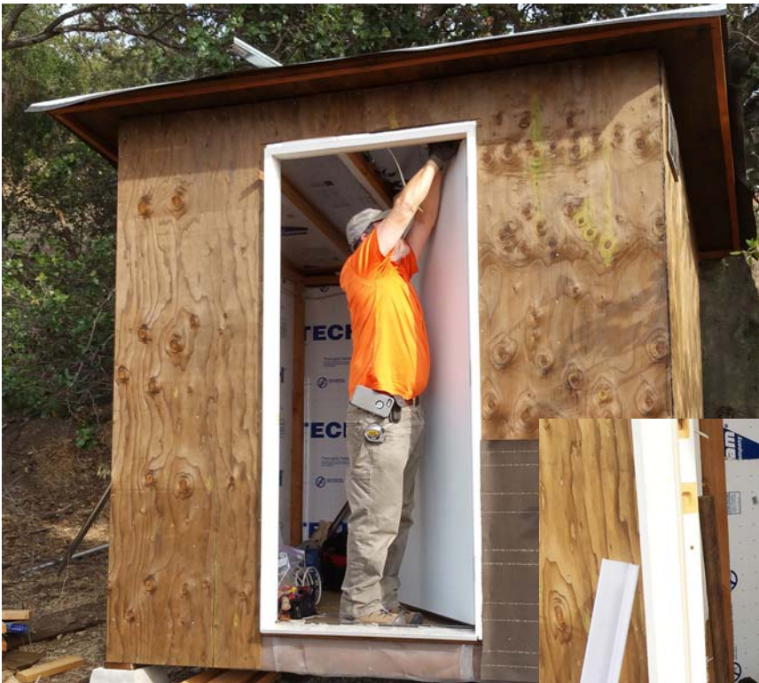
Jim K6SV installing a light fixture in the Repeater Shack
