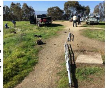
40 bolts had to be cut to take it apart
