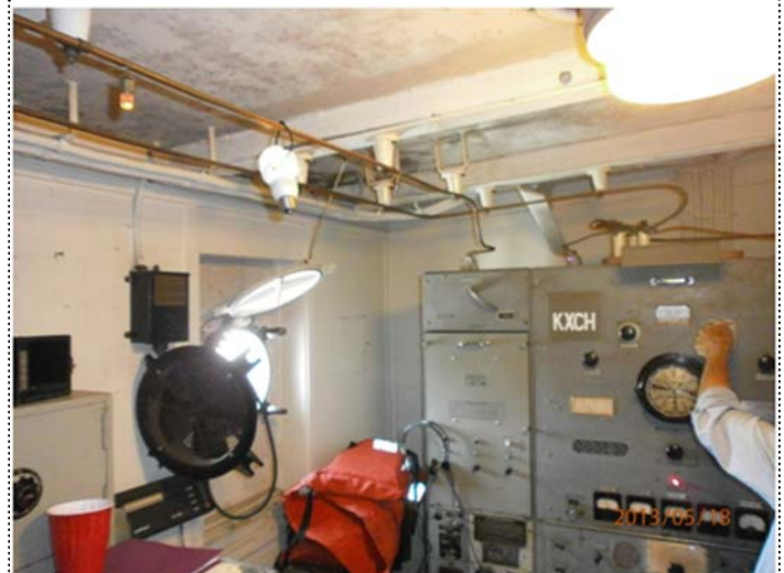
CFL hanging from the transmission line verifies we're transmitting RF.
