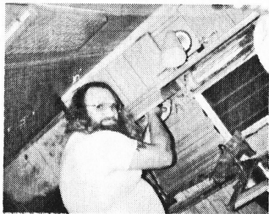
MIKE KD6EUD ripping out olde fixtures.
