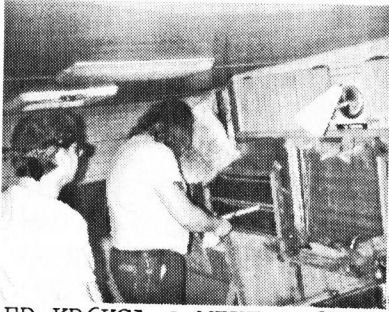
ED KD6KCA & MIKE KD6EUD, pulling out olde insulation.
